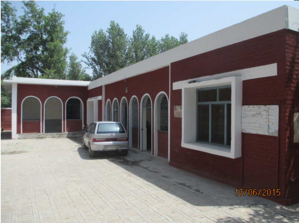
Figure 7: Rehabilitation of Basic Health Unit, Peshawar
