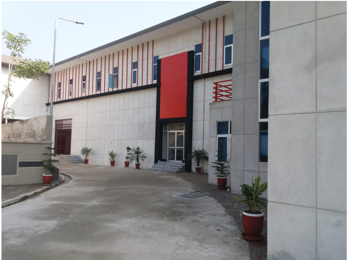
Figure 5: Construction of Provincial Cold Chain Warehouse – KP for the storage of children vaccines
